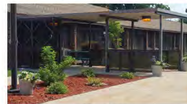
SHAWL I 225 South Hall Street in Whitehall
