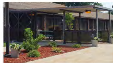
SHAWL I 225 South Hall Street in Whitehall
