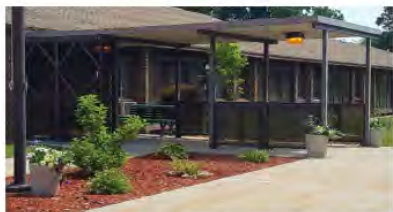
SHAWL I 225 South Hall Street in Whitehall
