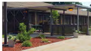
SHAWL I 225 South Hall Street in Whitehall
