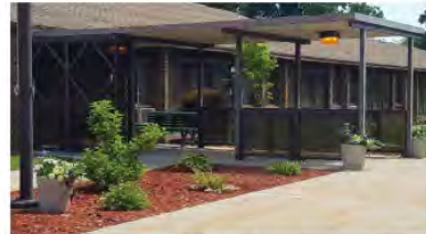
SHAWL I 225 South Hall Street in Whitehall
