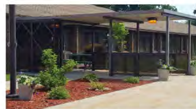
SHAWL I 225 South Hall Street in Whitehall
