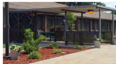
SHAWL I 225 South Hall Street in Whitehall
