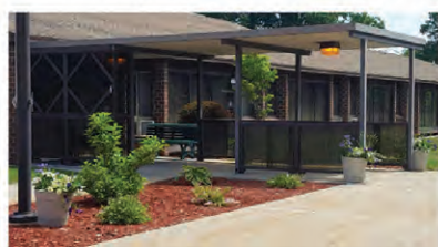
SHAWL I 225 South Hall Street in Whitehall
