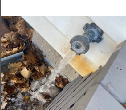
Exterior is functioning correctly
