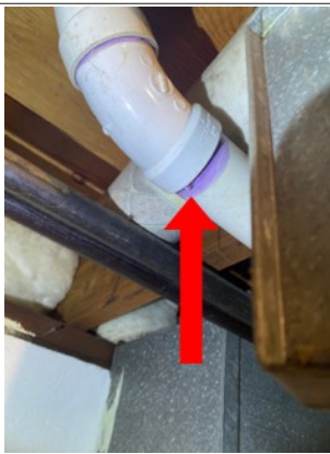
Condensation is dripping from the vent line. Recommend repair in resealing around this joint
