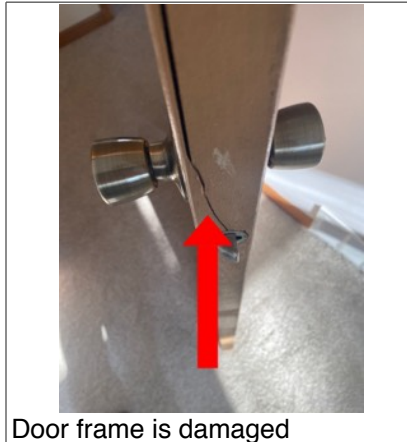
Door frame is damaged
