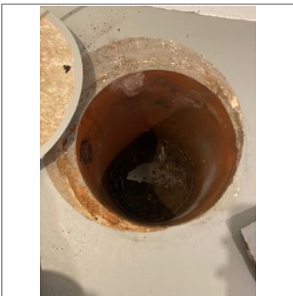
If water table rises, recommend installing sump pump
